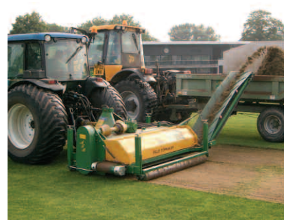
1. Planing off the surface to establish a primary level
