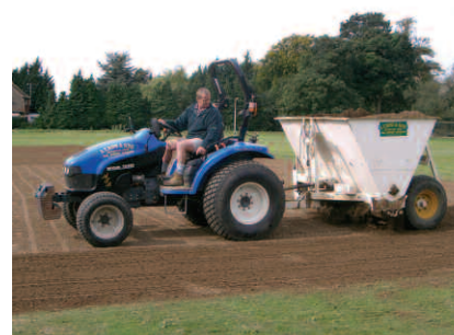
3. Spreading and integrating cricket loam
