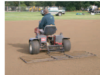
4. Grading to level
